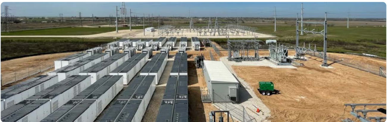
Two 50 MW BESS under construction in Texas, with a transmission substation in the background and a project substation on the right. (Photo: Key Capture Energy)
